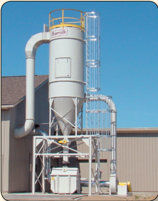
EFR Cyclone filter combination on a sub-stand with a Lacey Harmer dumpster under for storage.
