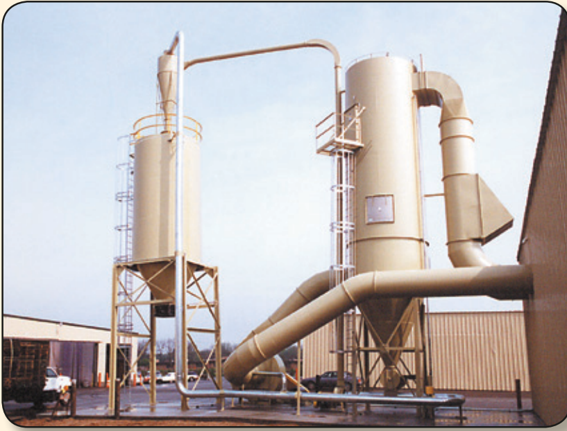
Relay cyclone on top of a Honeyville Metal welded storage bin with overhead load-out. Cyclone is one component in this complete Honeyville Metal Dust System in a woodworking plant.
