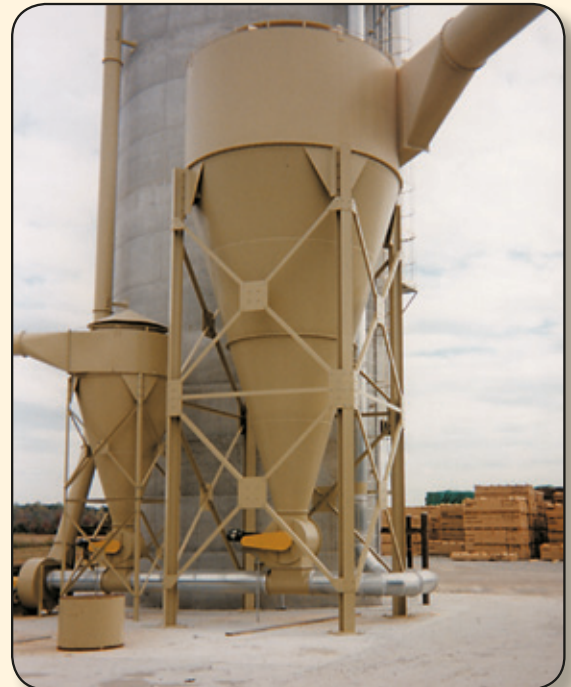
Two open top cyclones dropping into a common closed loop relay system.
